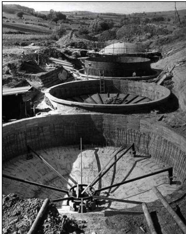
Figure 12. Liquid waste tanks during construction
