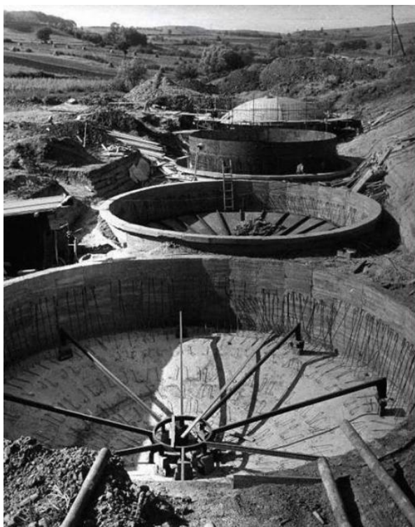
Figure 11. Liquid waste tanks during construction
