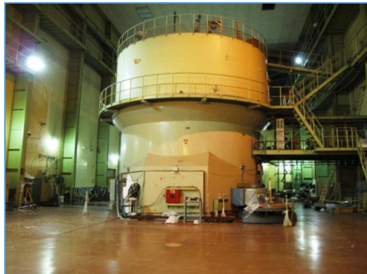
Figure 2. RA Research reactor
