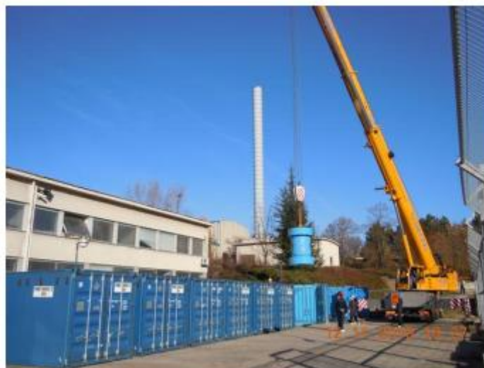
Figure 42. Loading of the ŠKODA cask into ISO container
