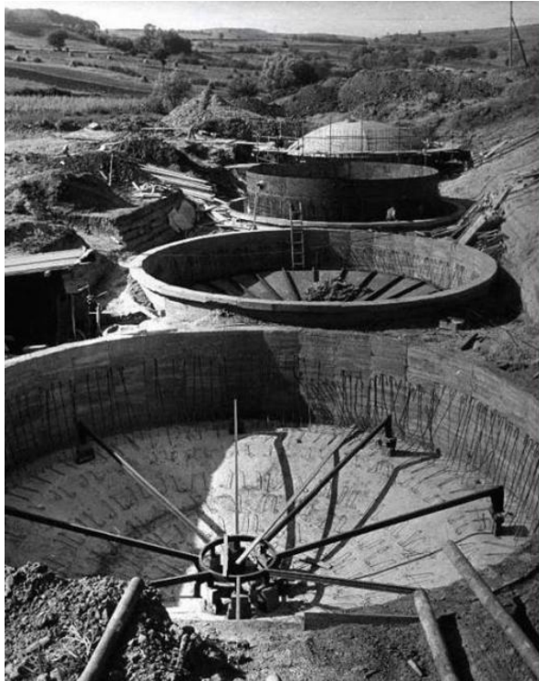
Figure 22. Underground liquid waste tanks during construction
